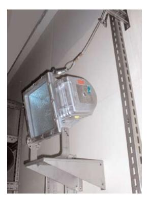
Many floodlights installed at height are not adequately secured against falling or colliding with mobile equipment.
